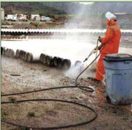
Here is an example of water blasting pipes using VpCI™-611 to protect the uncoated surfaces.
